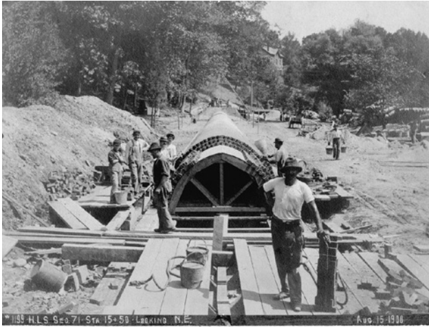
The 9-foot-diameter sewer line being installed in Bussey Brook Meadow in August 1900.
